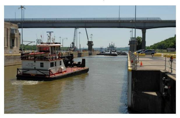
The Markland Locks & Dam is located on the Ohio River. It is 26.5 miles upstream from Madison, IN and 3.5 miles downstream from Warsaw, KY. The navigation locks are located on the Kentucky side of the river. The upper pool above the dam extends upstream for a distance of 95.3 miles to the Meldahl Locks and Dam.
